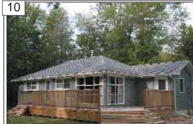
10 KINCARDINE, ON Year round home or cottage. This home has just been moved to this location and features a brand new foundation and septic system. Total open concept main floor with kitchen, dining and living room. Large private lot close to the beach
