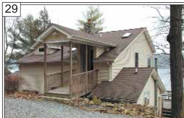
29 MILFORD, NJ Great Lakefront Home on Greenwood Lake. Private Location, Amazing Lake Views, 150 Feet Lakefront, 2 Decks, 2 Docks, Tons of Windows, Hardwood Floors and Much More!
